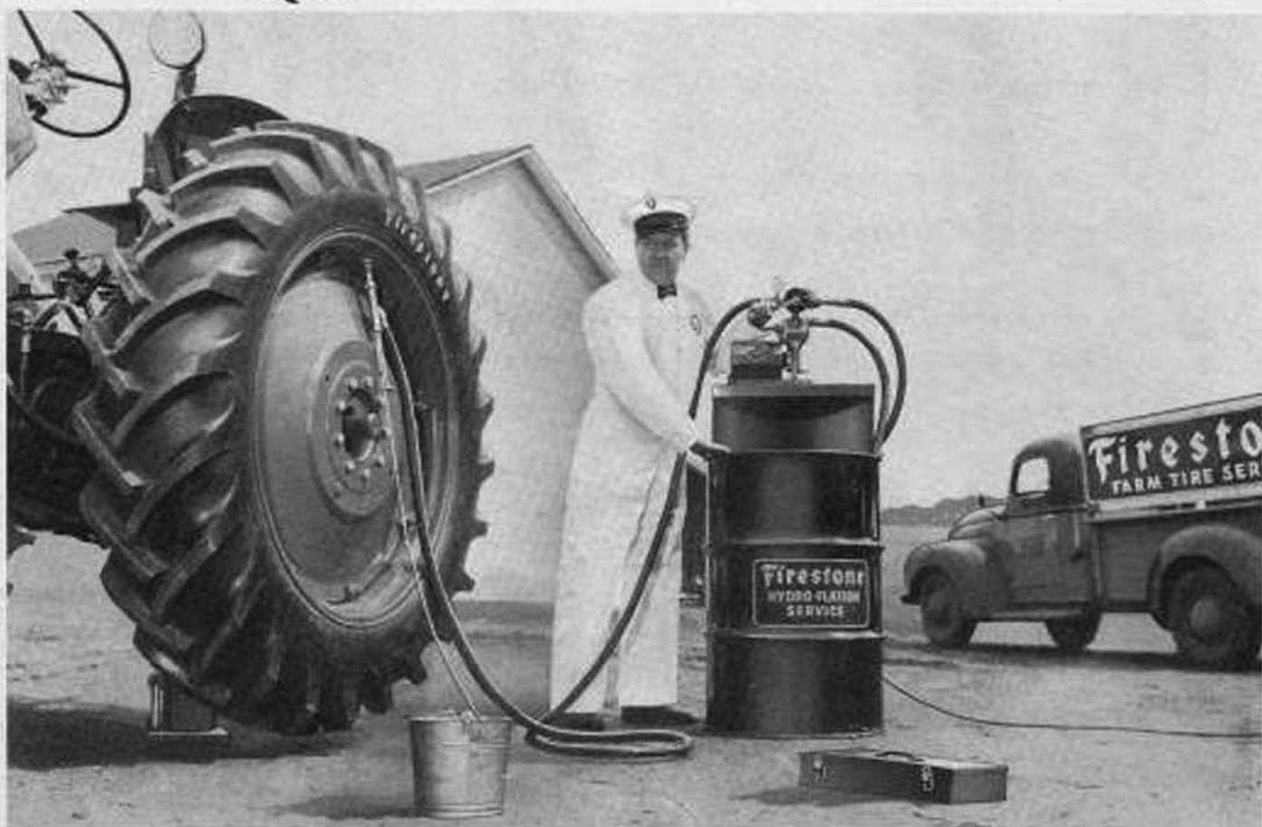
Operating a Firestone electric Hydro-Flator on a farm.
